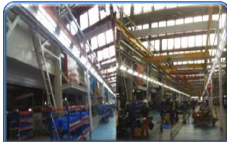
New energy efficient 40W LED Batten lights
