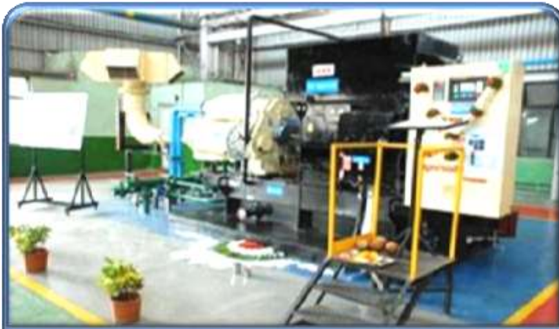
3000CFM Energy Efficient Centrifugal Compressor IR make Installed
