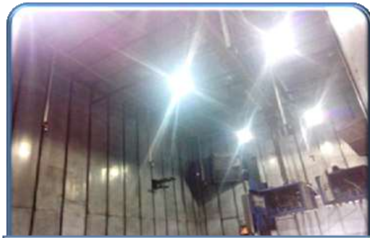
Installation of Flameproof 30W Energy Efficient LED Lights
